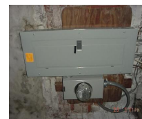
Major Systems Repair
